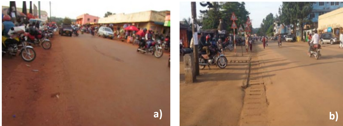
Figure 4. a) Unpaved and Dusty Walkways Near the Bus Terminal Encroached by Motorcycle Parking and Informal Trading, Obstructing Pedestrian Movement; b) Paved and Demarcated Walkways along Kashozi Road Shared between Pedestrians, Informal Trading, and Motorcycle Parking
