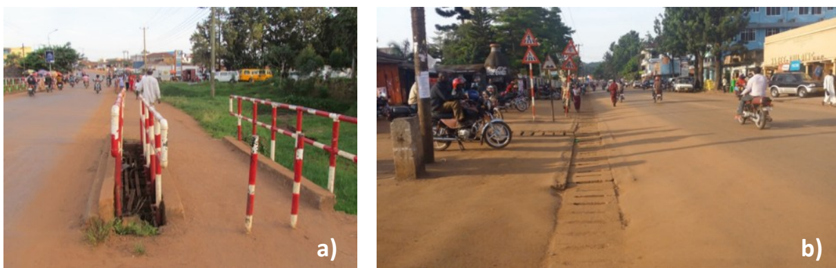
Figure 7. a) Pedestrians' Path on the Bridge Secured with Side Rails; b) Natural Trees, Traffic Signs, Billboards, and Covered Storm Water Drainage Channels as Basic Street Furniture and Facilities
