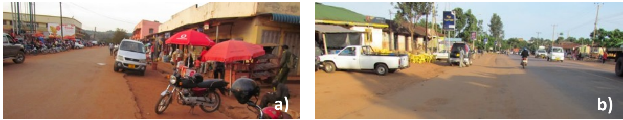
Figure 6. a) The Mix of Buildings, Informal Parking of Cars and Motorcycles, Displays of Petty Traders' Goods, and Makeshift Huts Affecting the Architectural Character of the Urban Street; b) Buildings along Uganda Road in the Hamugembe Area, Predominantly Single-Storey Structures Occupied by Commercial Functions
